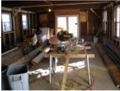
Education Room under construction.
